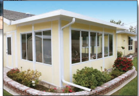
Custom painted exterior walls to match house.
